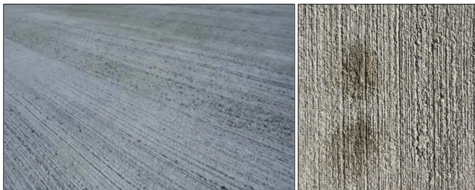
Image 2: Concrete Surface Brushed with a Broom
